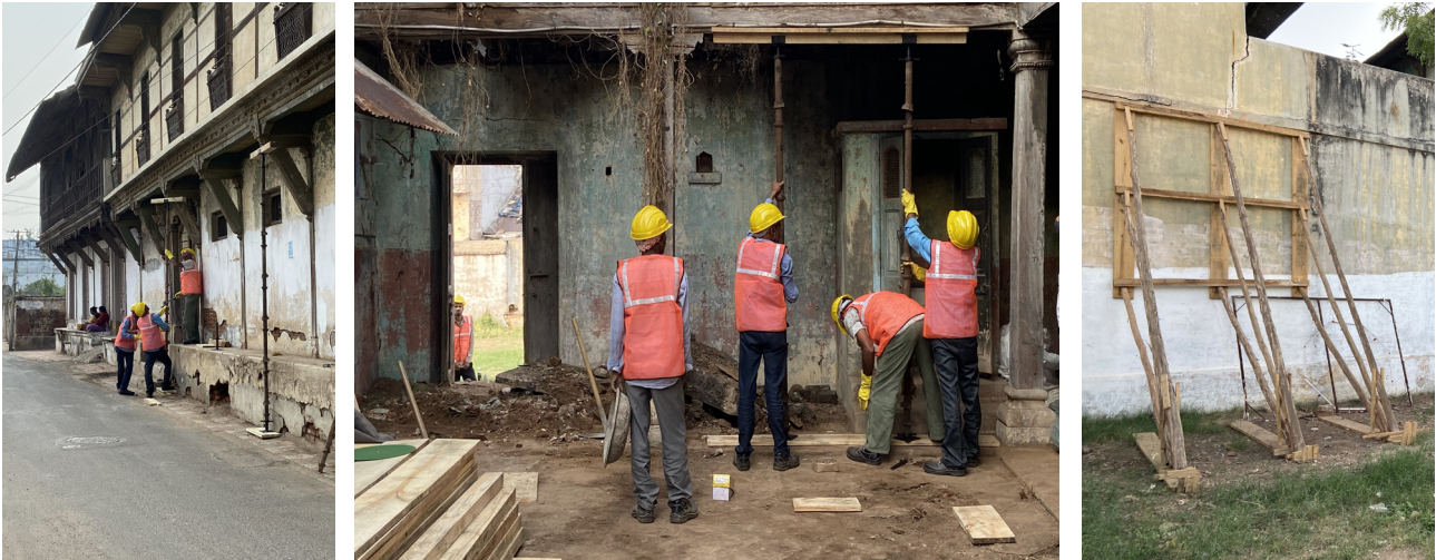
Propping up of timber beams and shoring of the side wall of the front wing of Kalidas Jethabhai House
