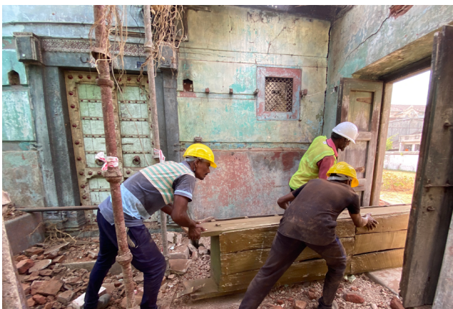
Segregation of construction material, timber elements and debris, Source: CHC, CRDF
