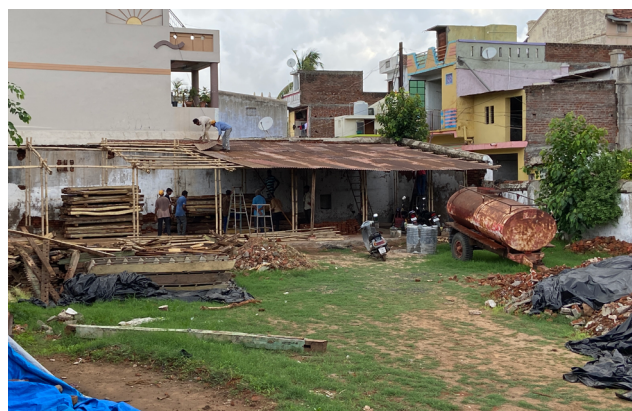
Material shed construction for storage of recovered material, Source: CHC, CRDF
