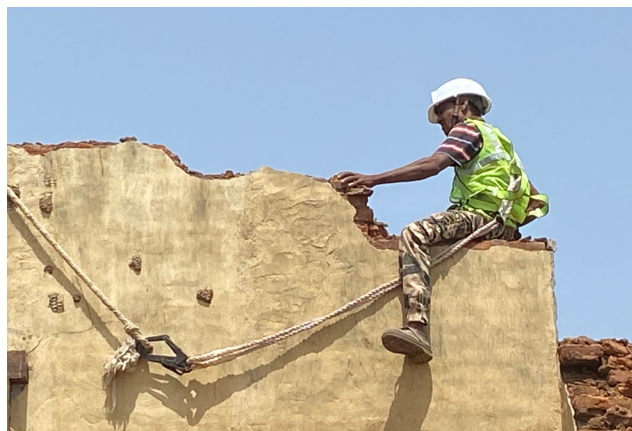
Floor-wise dismantling of the back wing with appropriate safety measures, Source: CHC, CRDF
