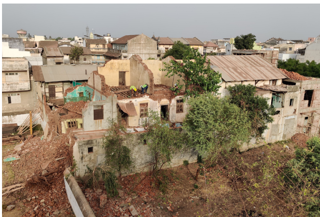
Floor-wise dismantling of the back wing with appropriate safety measures, Source: CHC, CRDF
