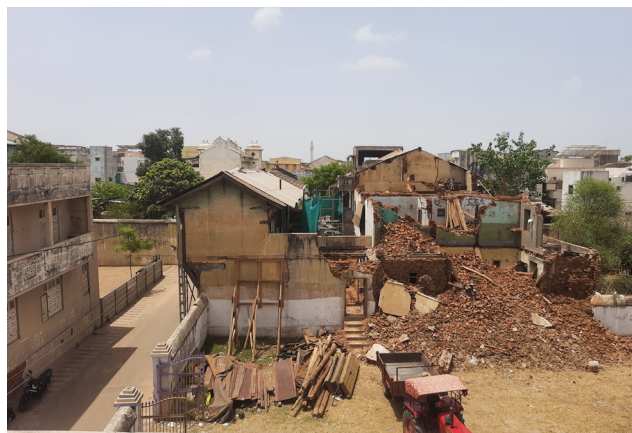
Segregation of construction material, timber elements and debris, Source: CHC, CRDF
