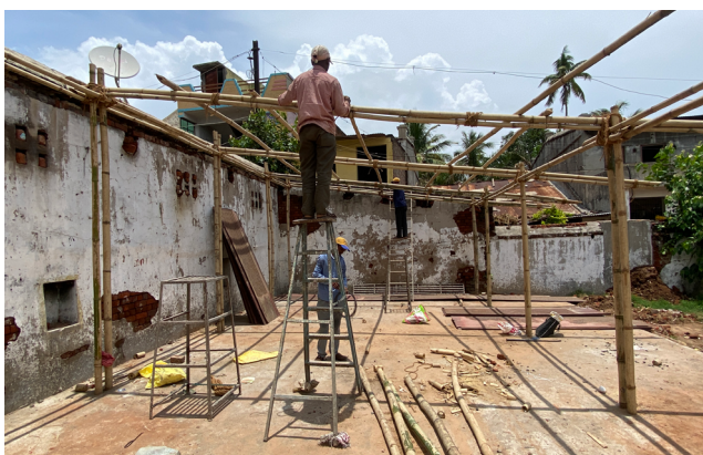
Material shed construction for storage of recovered material, Source: CHC, CRDF
