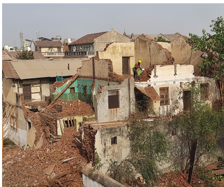
Careful dismantling of the back wing of Kalidas Jethabhai House (photographs by Audrey Alvares)
